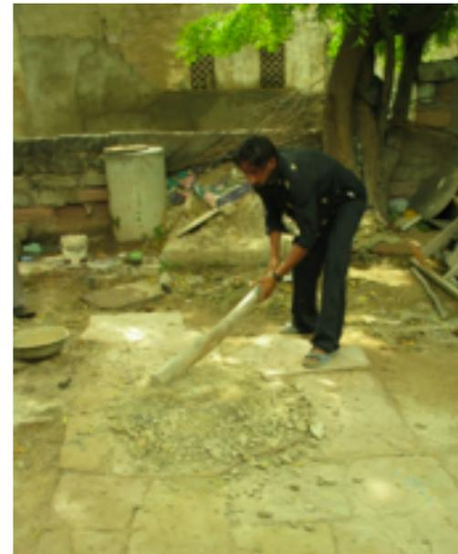
Breaking chunks of clay to sieve.
