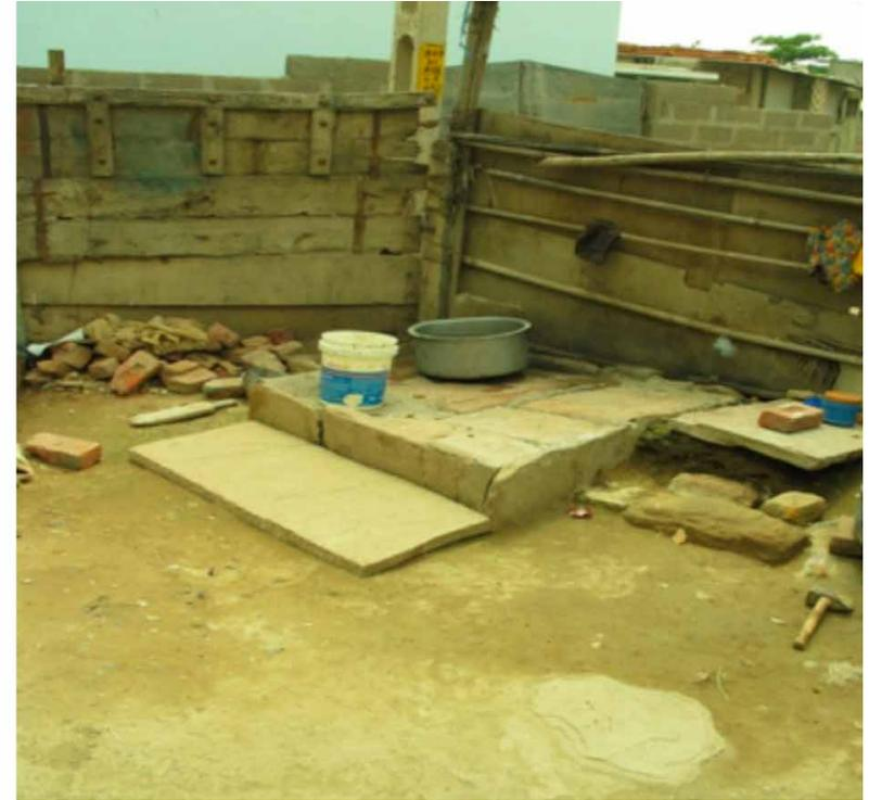
Clay is soaked in shallow pits for a couple of days and wedged on the cemented area
